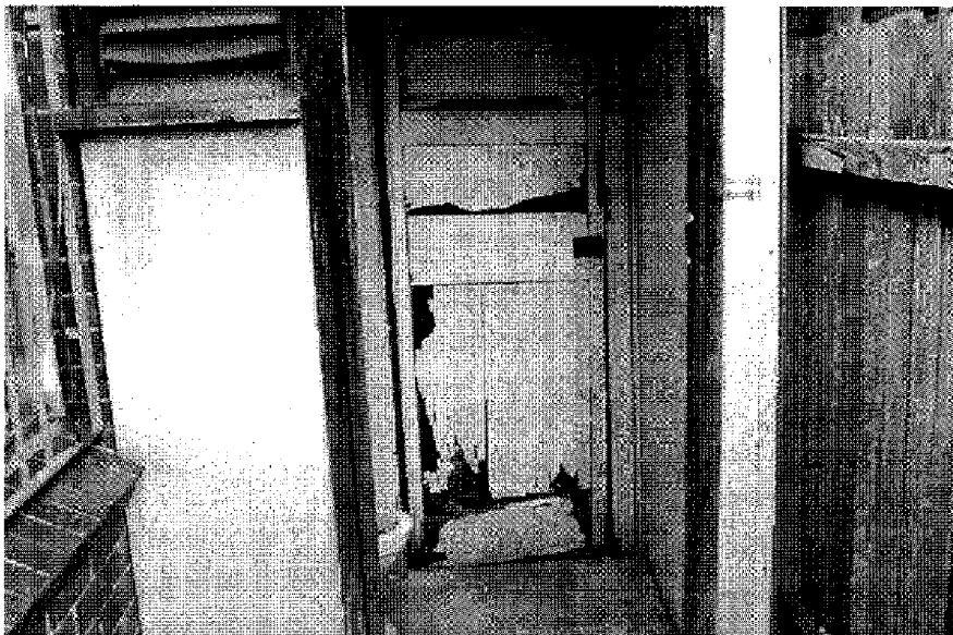
Photo 17: Asbestos cement sheeting located in the ceiling and internal and external wall cladding of the outside toilet of residential tenancy at 89C Liverpool Road. Also shown is white paint with elevated levels of lead.
