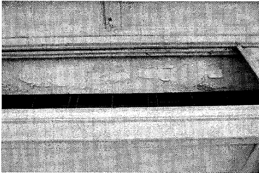
Photo 7: White paint with elevated levels of lead on the lintel and ceilings of the commercial tenancy at 89 Liverpool Road.
