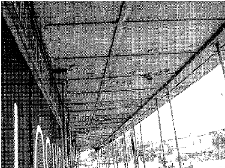
Photo 1: Asbestos cement sheeting located on the underside of the street awnings. Also shown is flaking white paint containing elevated levels of lead.
