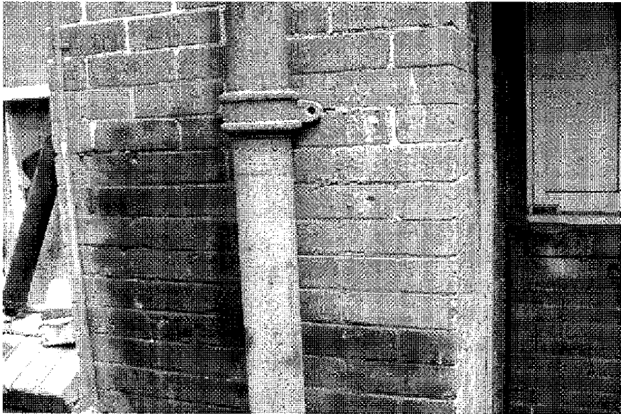
Photo 33: Red paint with elevated levels of lead located on the drainpipe at the rear of residential tenancy 91B Liverpool Road.
